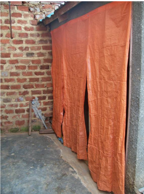
These are the ladies toilets at the school. The one on the far end is for the school staff and guests.
